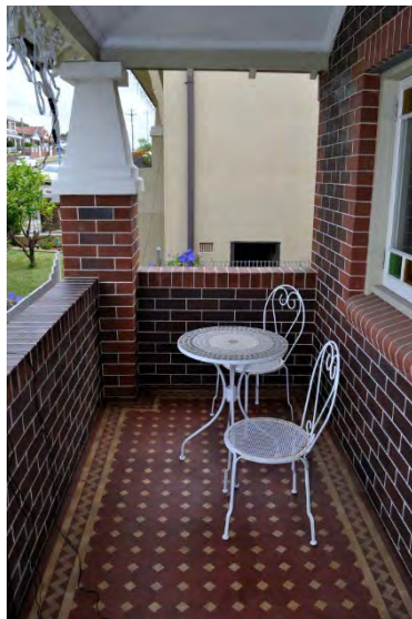
4. Verandah- tessellated tiles.
