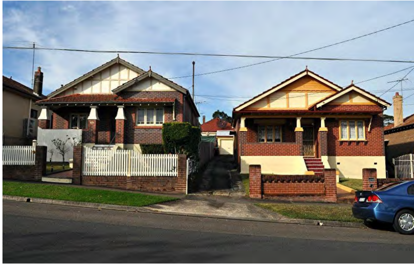
2. Subject property (LHS) and adjoining house No 42.
